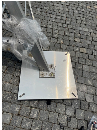
Fig. 9. Affixing the tower to the base
