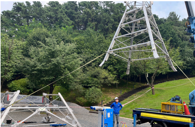
Fig. 8. Securing the base to the ground
