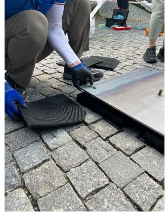
Fig. 7. Leveling the bases
