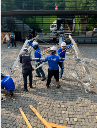
Fig. 5. Assembling the lower frame of the main tower
