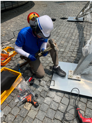
Fig. 8. Securing the base to the ground
