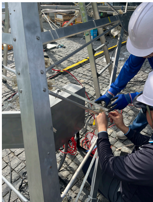
Fig. 14. Installing neon tubes
