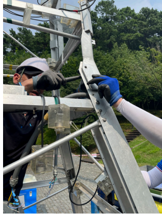
Fig. 6. Connecting the sides of the lower and middle frames
